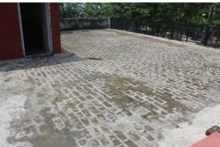
The school building was old with an old-style brick roof. Lack of any infrastructure upgrades over the past many years had led to damage. This posed a threat to the interior repair that was done in the previous year as the roof would leak during monsoons and damage the interiors as well.
